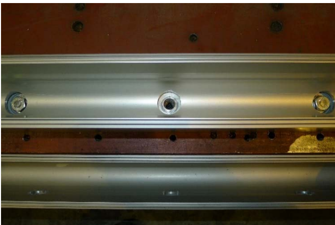
Figure 2 typical bolt fixtures at 400mm centres.
